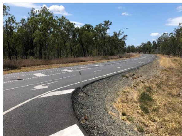
Figure 6 South on Bruce Highway from South Ulam Rd
