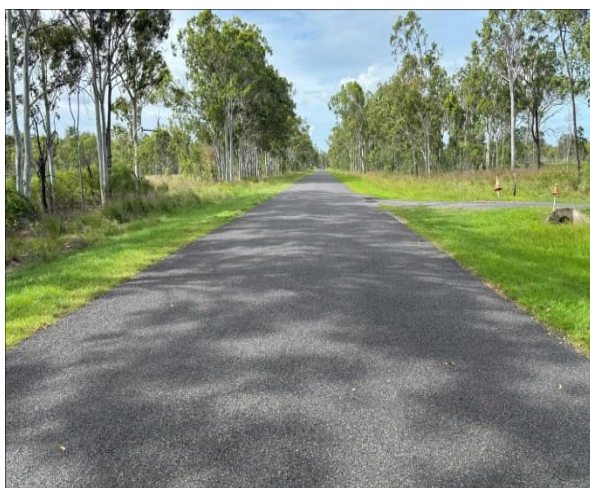
Figure 3 Northern End of South Ulam Road
