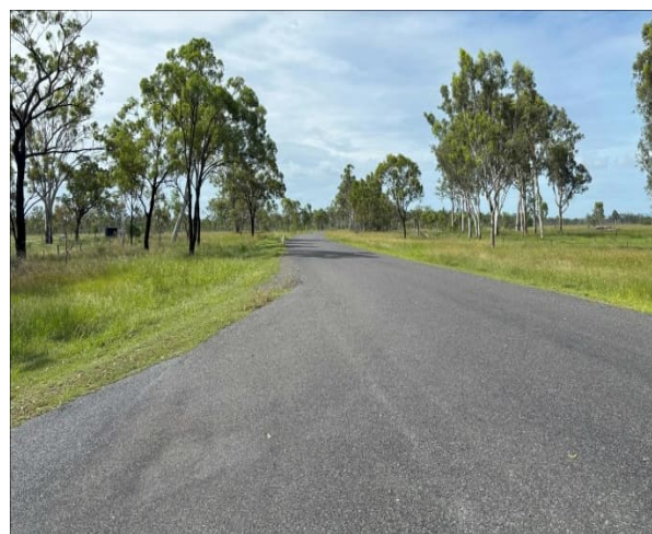
Figure 4 Southern End of South Ulam Road
