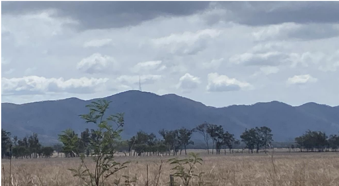
Figure 10 Existing telecommunication tower, view from South Ulam Road
