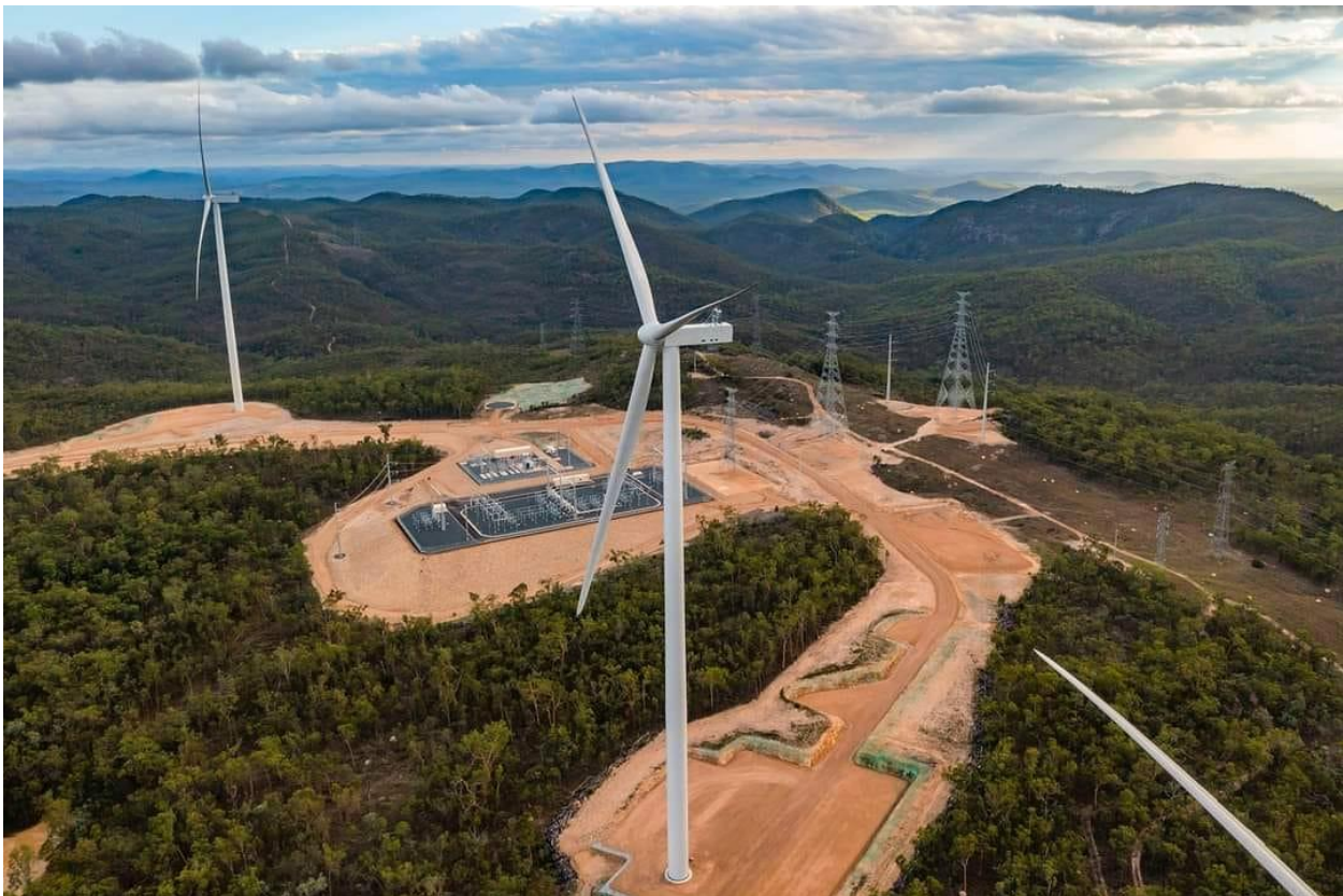
Image - habitat destruction for Kaban wind development, FNQ
