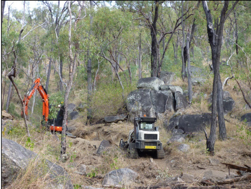
Photo 4: Recontouring access tracks to support drainage paths post salvage.
